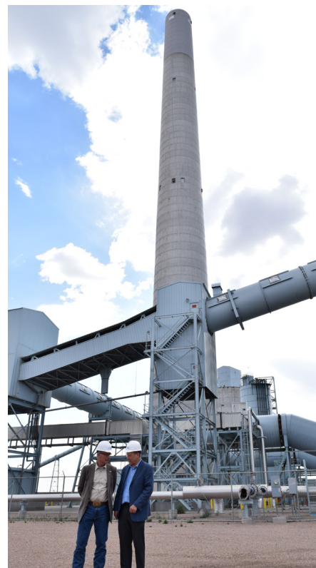
Wyoming Governor Mark Gordon stands in front of the Dry Fork Station just outside of Gillette, Wyoming, where the state tests carbon capture technology. Several of the policy recommendations in his WGA Chair initiative, Decarbonizing the West , were adopted by Congress this year.
