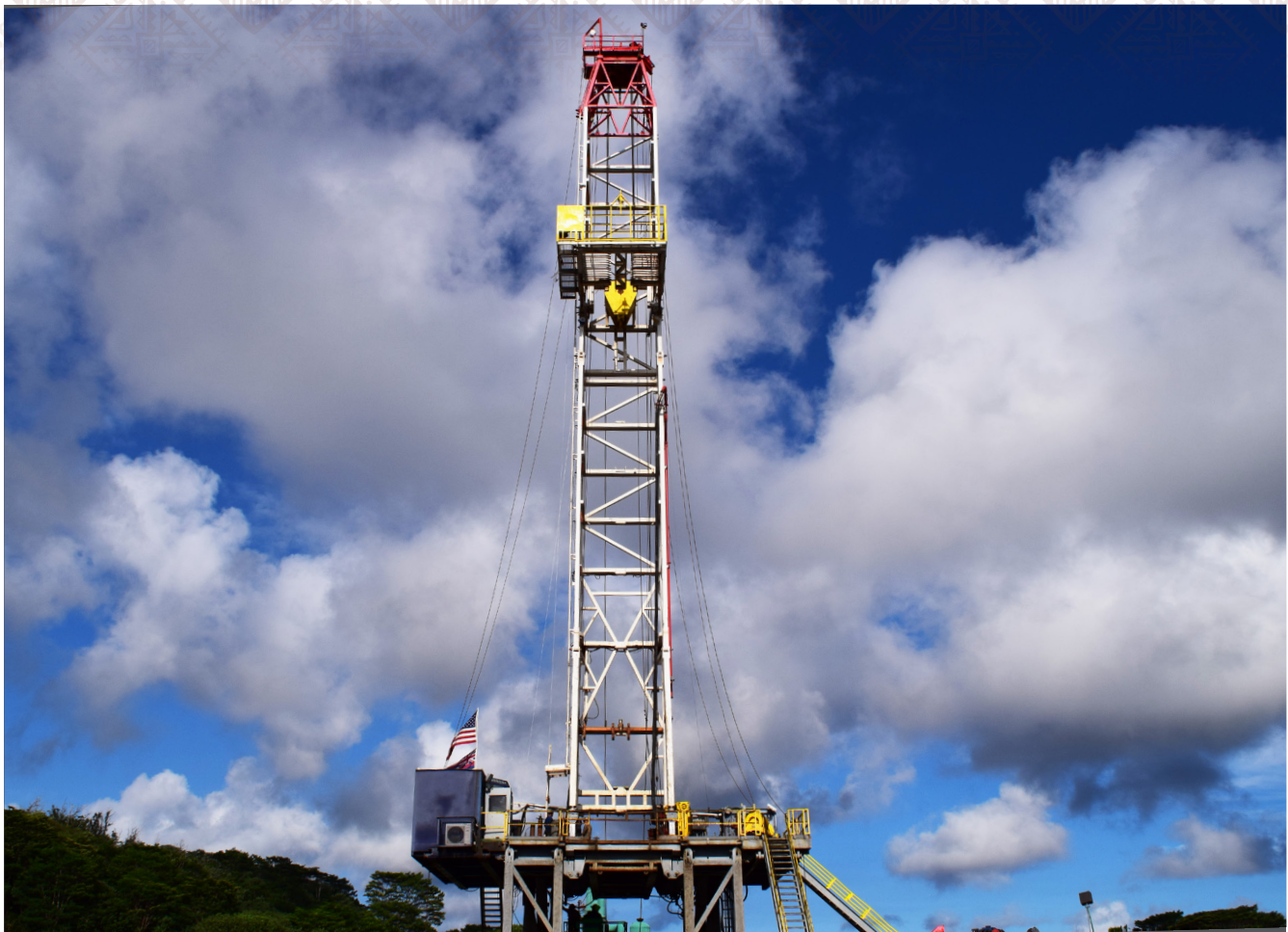
Preparing for drilling at the Puna Geothermal Venture, operated by Ormat Technologies Inc. The exploration and drilling phases often bring the highest risk for failure and the most cost to geothermal development.
