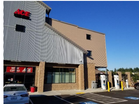
DuPont Ace Hardware (2 DCFC, 1 L2 EVSE)
