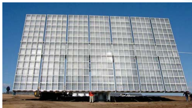
Concentrating photovoltaic cells, such as this array in Arizona, help the West take advantage of its vast solar resources. Photo Courtesy NREL/Pix - Robert McConnell
