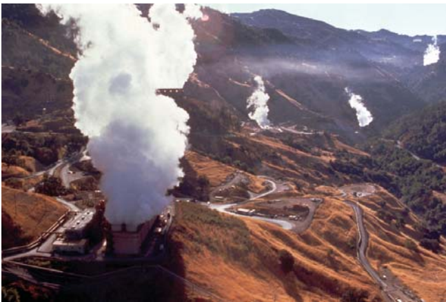
The largest geothermal field in the world is The Geysers, near San Francisco. Photo Courtesy NREL/Pix - Pacific Gas and Electric
