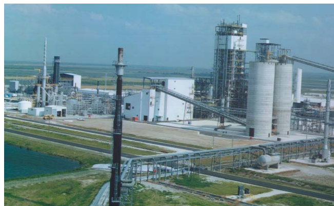
Advanced coal technologies, such as IGCC, will help electrical generation from coal move towards near-zero emissions. Photo courtesy of U.S. DOE.
