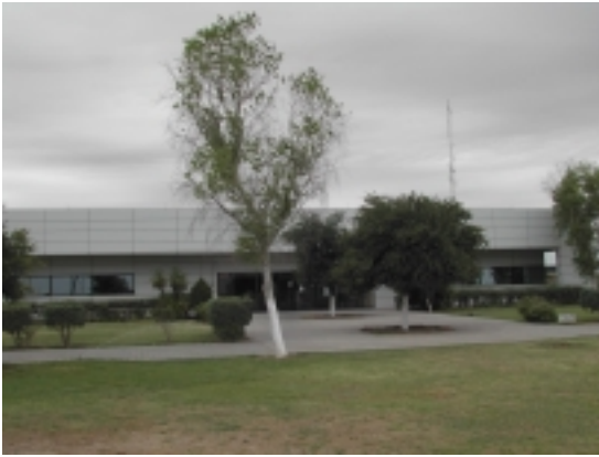
Figure 11. Aduana Colombia Offices
