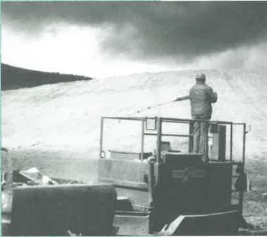
Workers seed a tailings pile at a Colorado mine.
