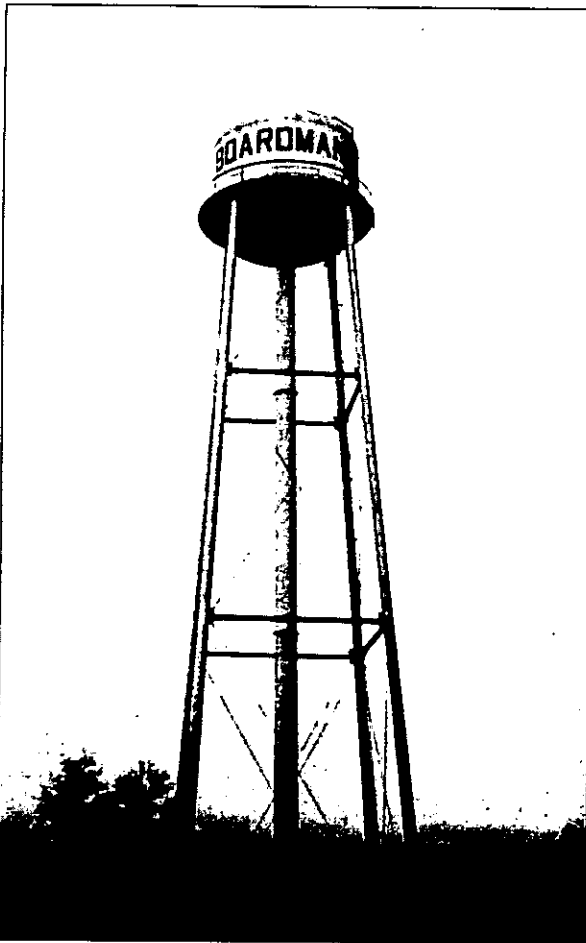
The Boardman drinking water system will need improvements to meet population growth and future requirements.
