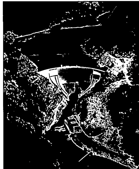
Dam on the Skagit River.
